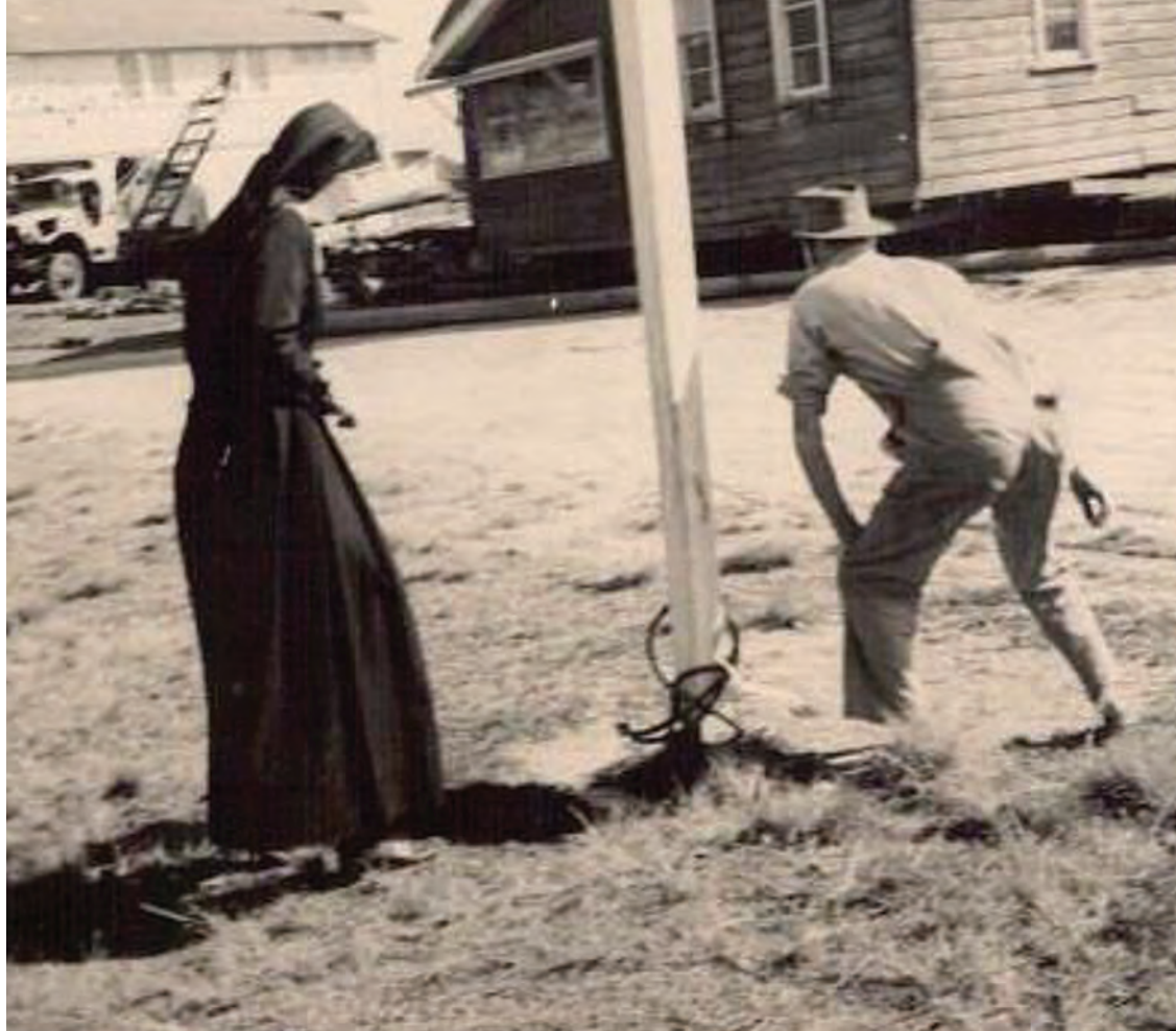
NUN AND BUILDER DURING WORKS ON ST FRANCIS XAVIER SCHOOL HALL
